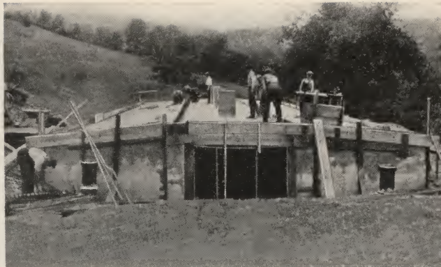
Nearly completed storage cellar with slightly arched concrete slab roof.
